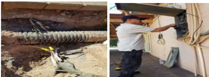
electricity line cut underground of temple
